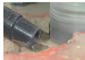
Vacuum drilling slurry
